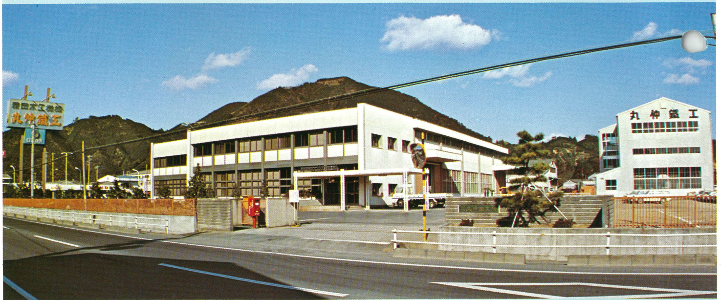
Entire View of Head Office
